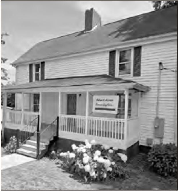
The electrical renovations are already finished, and the church is in the process of fundraising for plumbing.
